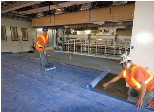
NobleSeal SIS offers the benefits of sound isolation, crack isolation and waterproofing, all in one sheet membrane.
