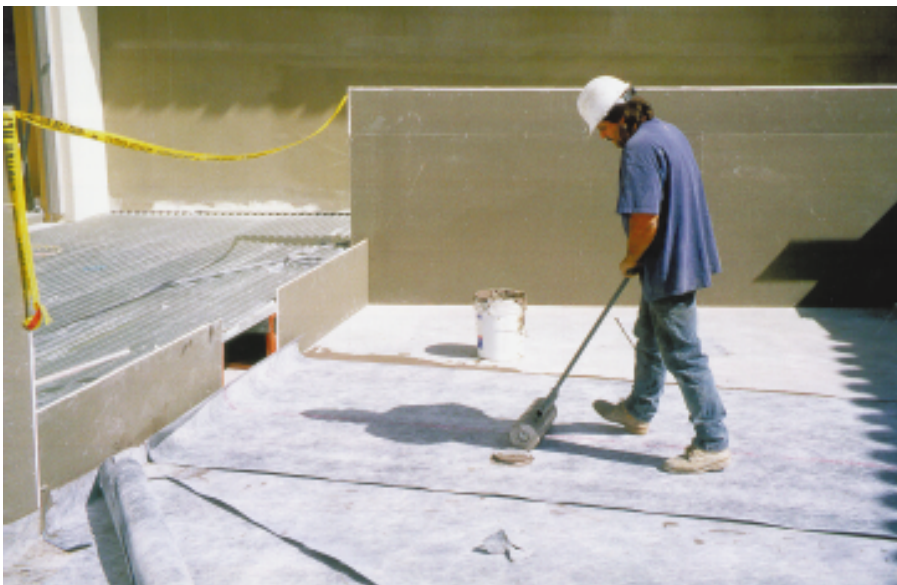
UV inhibitors and anti-oxidants are added to Noble Deck to guard against damage the sun could inflict on the membrane while exposed during installation.
