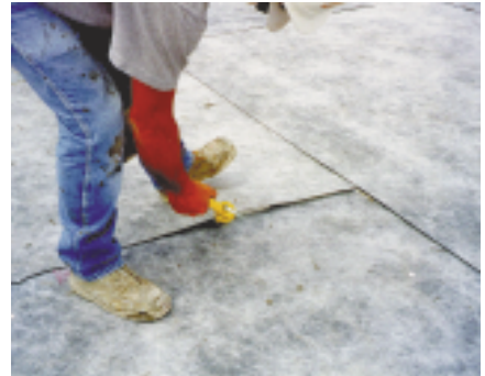
Use of NobleSealant 150 ensured quick, easy seaming for all overlaps.
