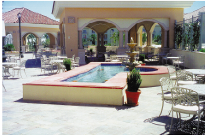
Noble Deck provided thin-set waterproofing for a complex, exterior installation.
