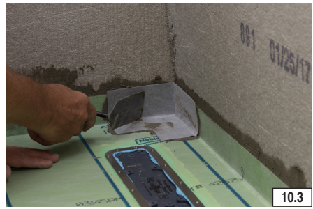
FIGURE 2: MEASURE AND CUT CURB WATERPROOFING
