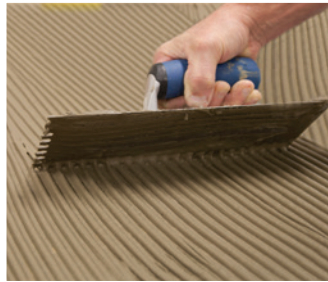
Apply thin-set to substrate
